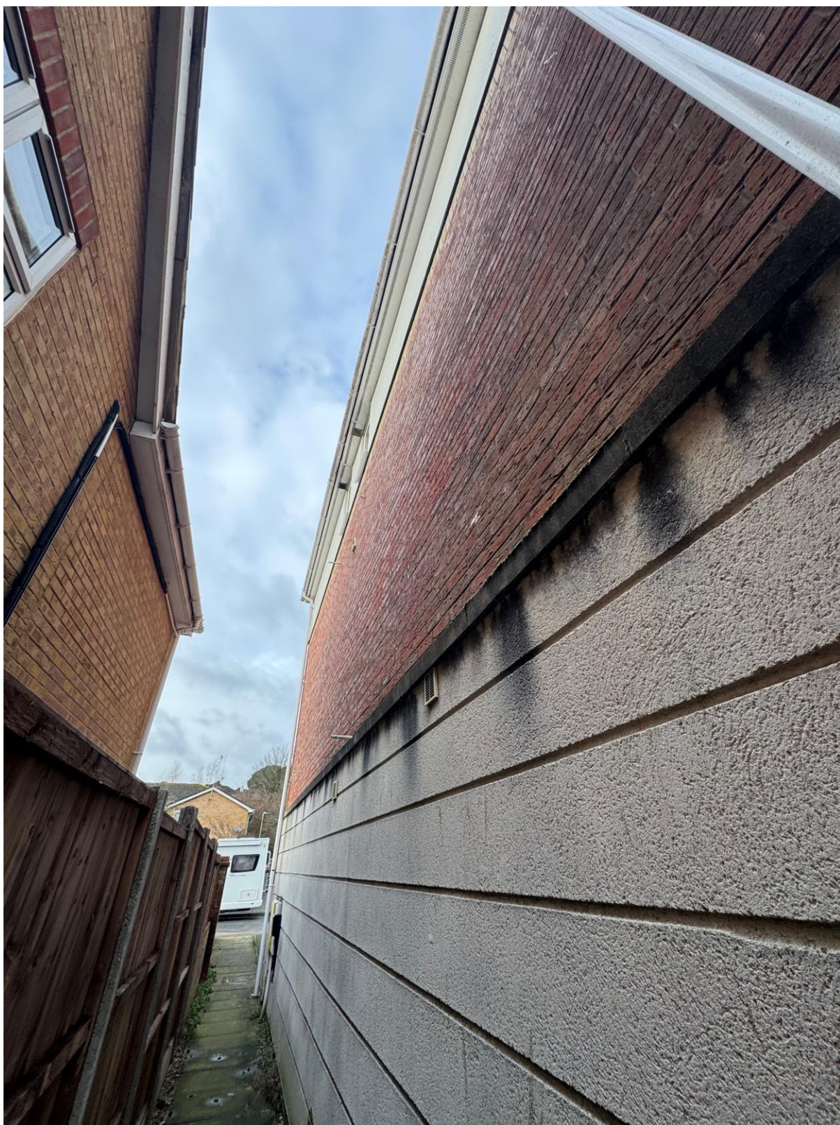
Figure 3: View of flank wall at ground level
