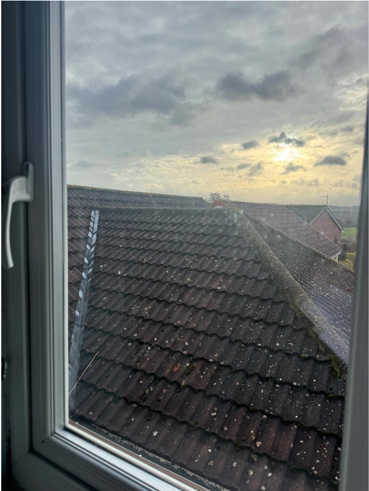
Figure 8: view from existing flank bathroom window at second floor level
