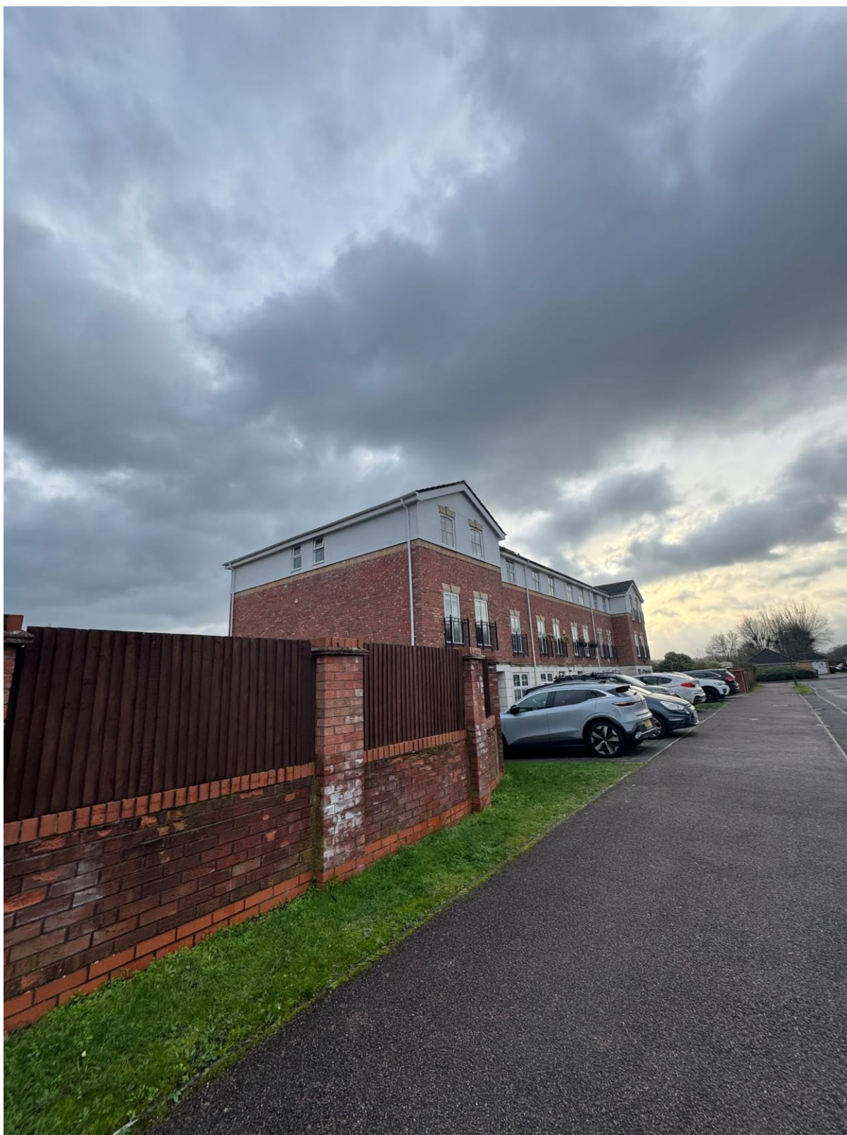
Figure 12: Flank elevation of No. 89 flank elevation with existing flank windows at second floor level
