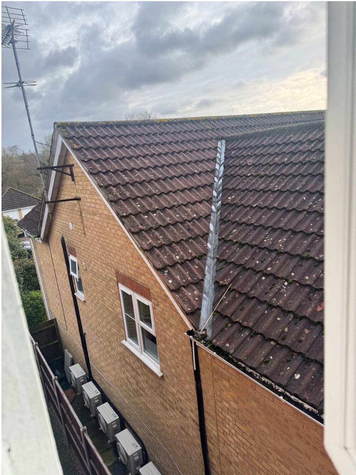
Figure 9: view from existing flank bathroom window at second floor level with window open
